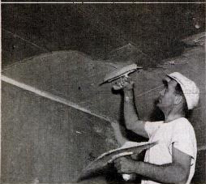
Photo above shows base coat of lightweight-aggregate plaster being applied. Ready-mixed avoids common problems of using bad sand or oversanding
